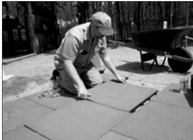
Playground Tile Installation
