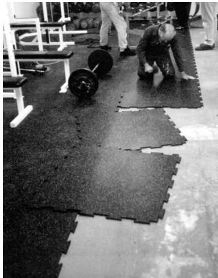
Four-Side Interlock Loose-Lay Installation
