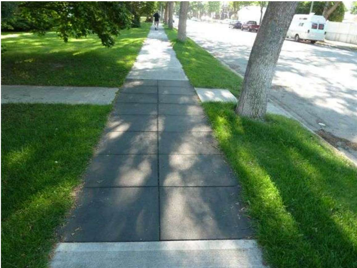
Rubber tiles along a sidewalk in Kelowna. (Contributed by Ian Wilson)
