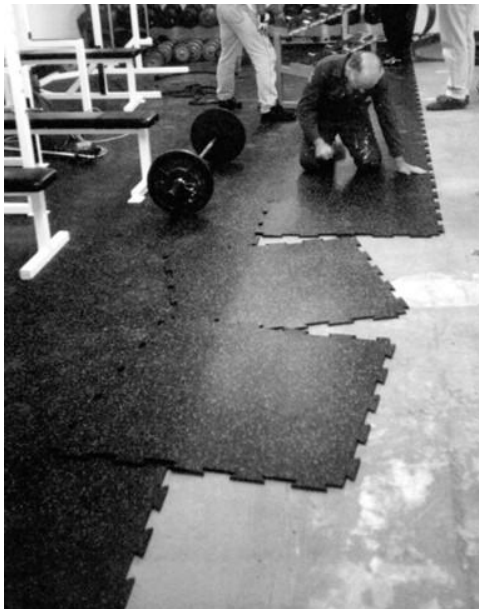
Four-Side Interlock Loose Lay Installation
