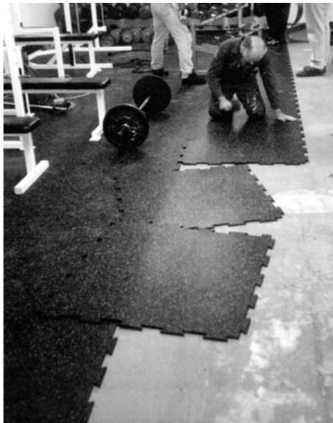
Four-Side Interlock Loose Lay Installation
