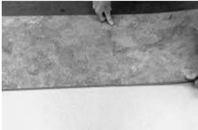
Square Cut Glue Down Installation
